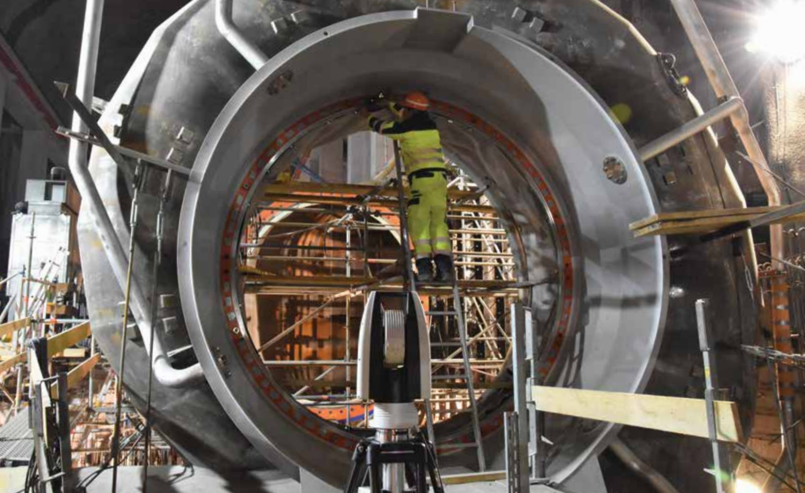
Before the reinforcement of its housing is cemented, the turbine spiral is exactly aligned with the Leica T-Probe.
